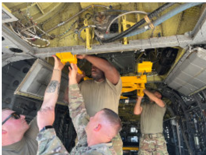
Reservists install the aft transmission (D. Lamere photo)
